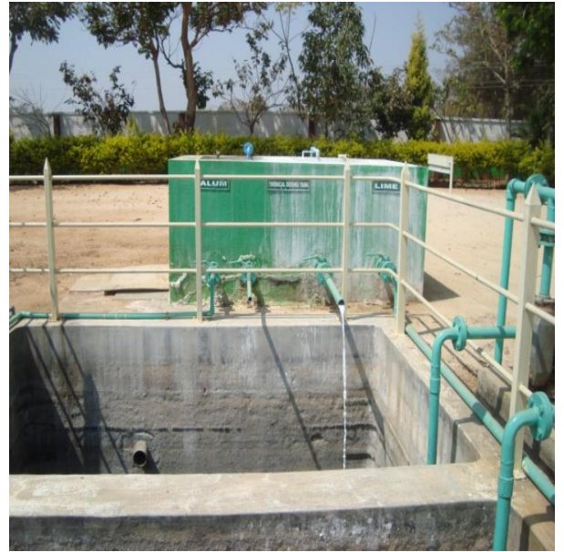
Fig 4 : Chemical dosage tank
