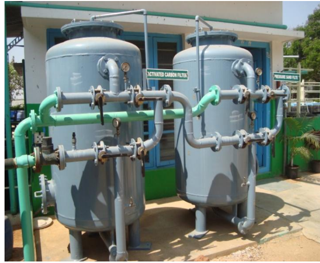
Fig. 8 : Pressure sand filter and carbon filter
