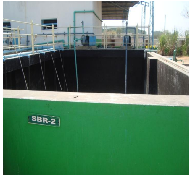
Fig. 6 : SBR-1 and SBR -2 for Low TDS effluent
