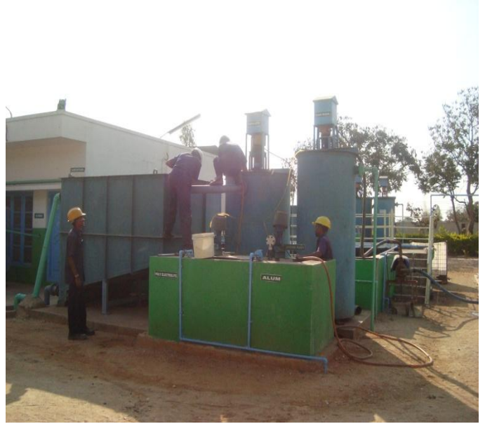
Fig 11 : Chemical dosage tanks, Flash mixer flocculator followed by plate settler (which was under repair during inspection)
