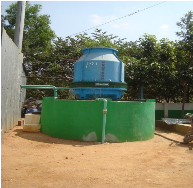
Fig 13. : Cooling Tower
