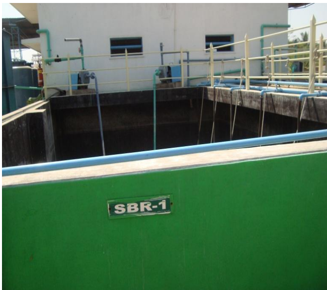
Fig. 6 : SBR-1 and SBR -2 for Low TDS effluent
