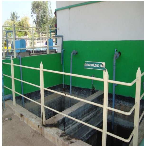
Fig 5. : Sludge storage tanks
