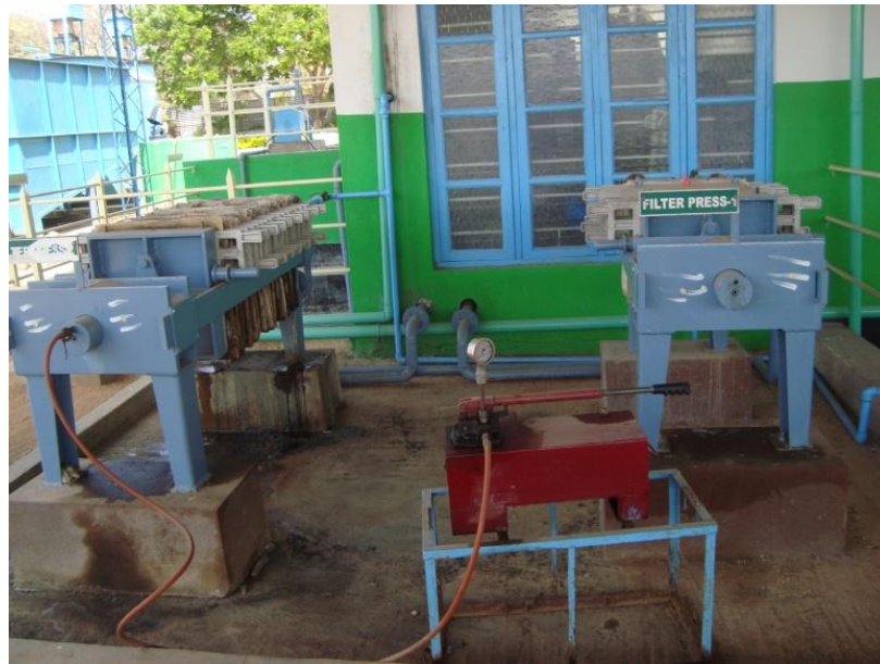
Fig 9. : Two filter Press to dewater the sludge generated from Low & high TDS chemical treatment, biological sludge and salt from MEE concentrate
