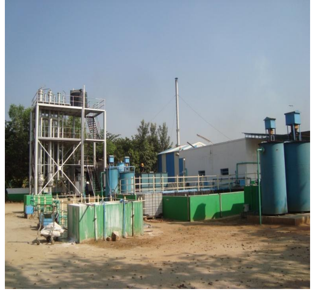
Fig 2 : Over all view of CETP
