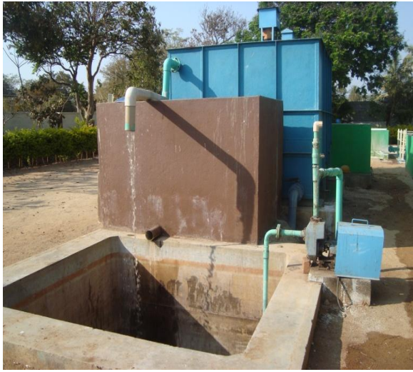
Fig. 7 : Treated water Collection tank
