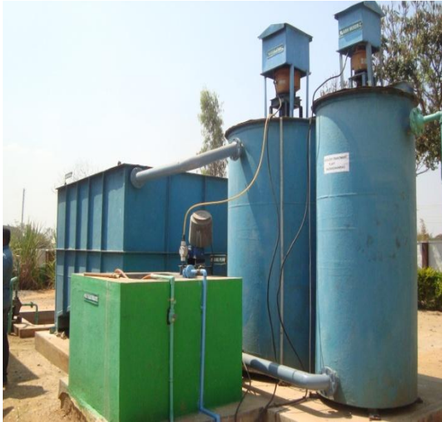
Fig. 4: Flash Mixer, flocculator followed by Plate Settler for Low TDS effluent
