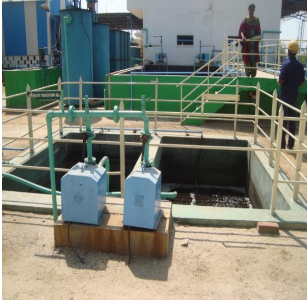
Fig. 10 : High TDS Collection tank
